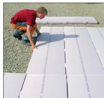
Utlegging Jackofoam® Sportsplate R+.
