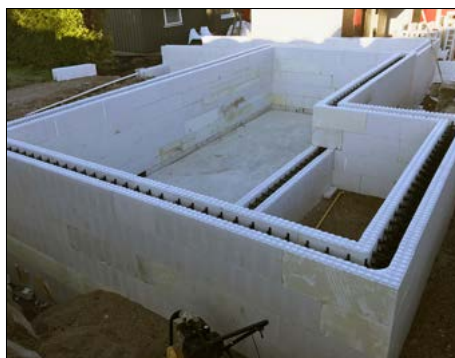
Jackon Thermomur® 250x Basseng uten tilbakefylling
